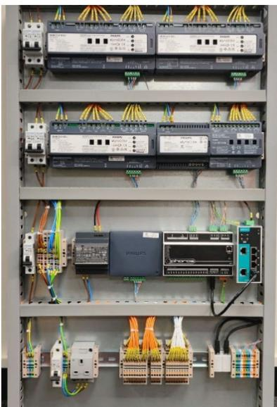
DIN rail mounted controllers
